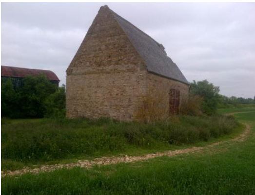
Photo 5: Barn C (North-west Aspect)
