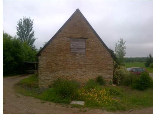
Photo 2: Building 1 (West Aspect)
