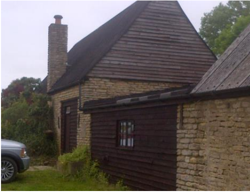
Photo 1: Building 1 (South-east Aspect)
