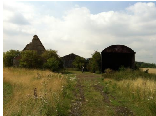
Photo 4: Barn B & C (South Aspect)
